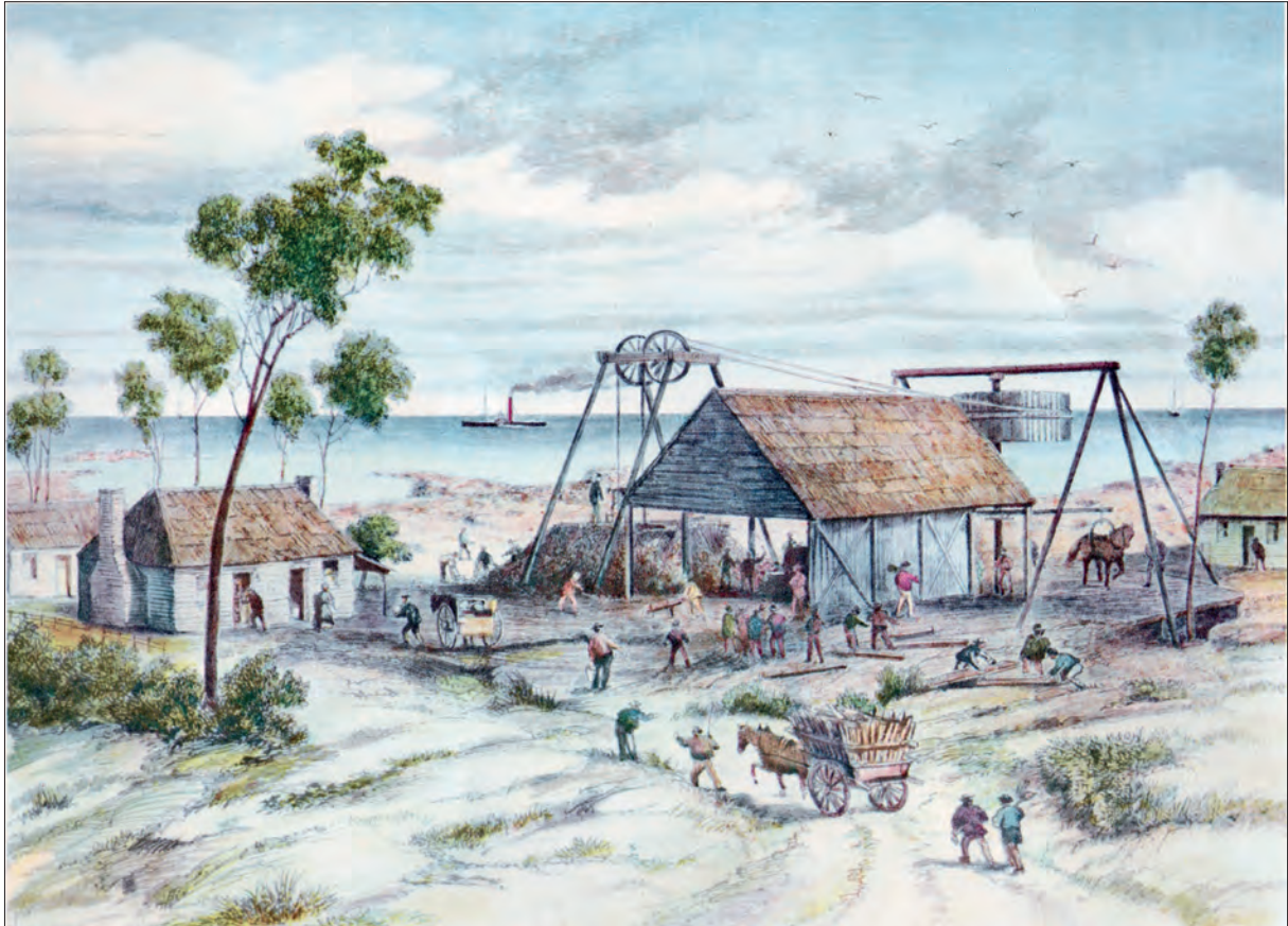
Further along the coast was the Penguin Silver Mine. Their beach-side operation was similar to the Tasmanian Copper Company, and this 1871 watercolour is also a good illustration of the operation of a whim for raising stone and water. In the background is the steam paddle tug Tamar.
