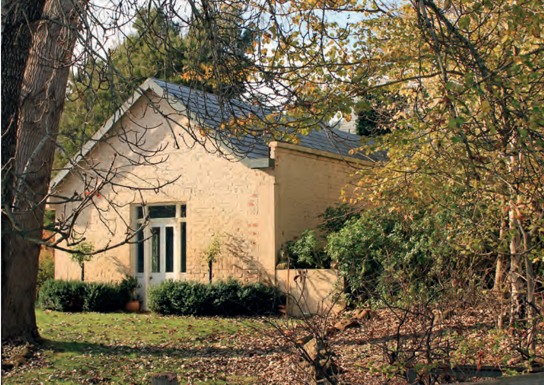
Above: The stone and brick residence next to Dilston Bridge—built by Captain George Coulson in 1838. It is often referred to as Dilston House. Image courtesy tasphotoalbum.com
