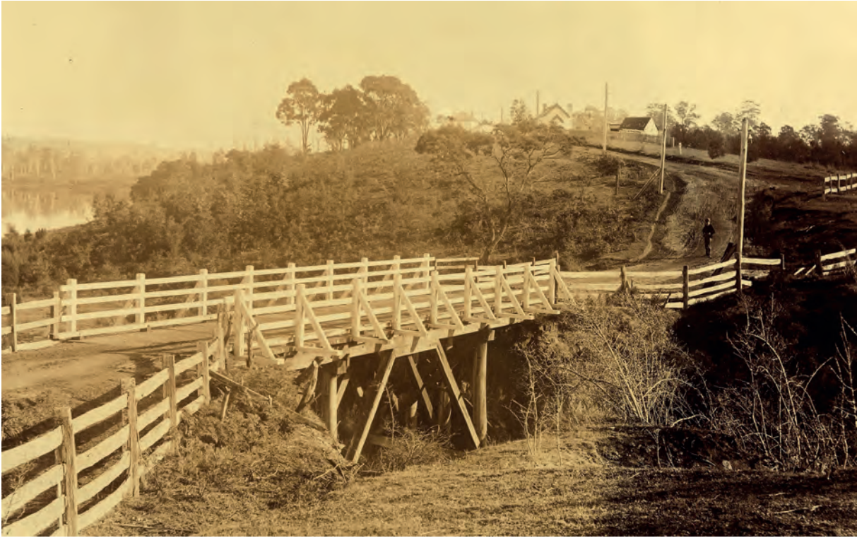
This c1898 photo is of the Dilston Bridge over the convict cutting that created Lady Nelson Creek. Dilston Church and hotel are in the background. Northern Tasmania Camera Club image courtesy TAHO.
