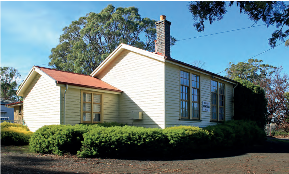
The Dilston School closed in 1953. The property had been earmarked for transportation to Ravenswood as a preschool, but was grabbed by the community, which needed a Memorial Hall. It was vested in Council in 1954 and administered by a local hall committee. That was also the year town water came to Dilston. Image courtesy tasphotoalbum.com
