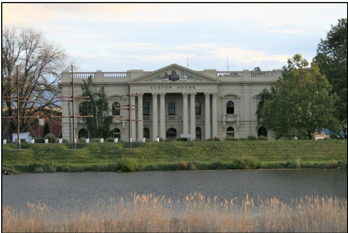
Custom House, Launceston, 87-89 The Esplanade protected by a flood levee: Ian Pattie photograph 22 Oct. 2020. Note: ship's masts installation
