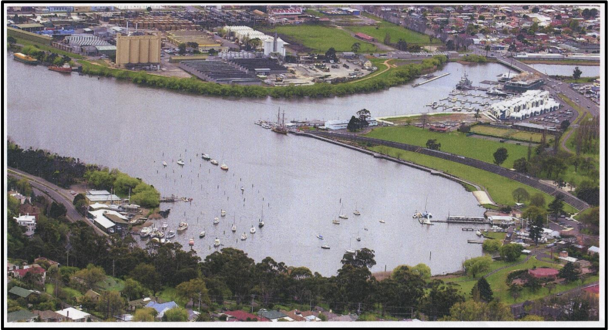
High tide in Launceston 9 October 2003: Launceston Examiner picture, showing the concrete flood training wall, built in the 1960s
